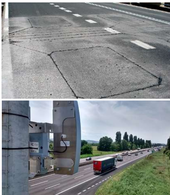
Figure 4 – Examples of intrusive and non-intrusive (Bluetooth) sensors. Lower image courtesy of Traffic Now
